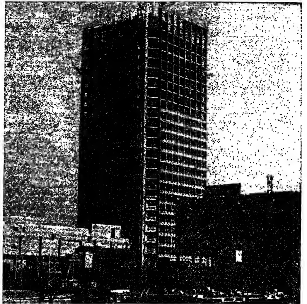
The Dubai International Trade and Exhibition Centre project, being constructed by Bernard Sunley and Sons.
